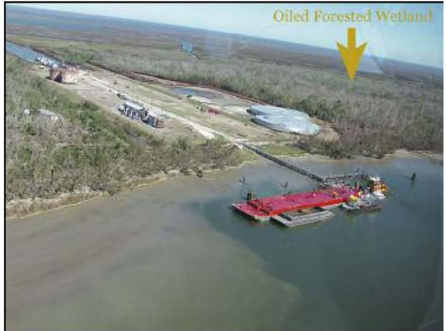
Figure 2: Oil from damaged tanks was moved by hurricane forces into impassable forested wetlands. USCG photo.
